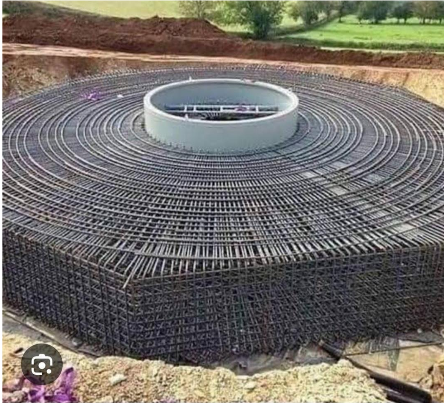
The amount of steel in a wind turbine footing. : r/Concrete
