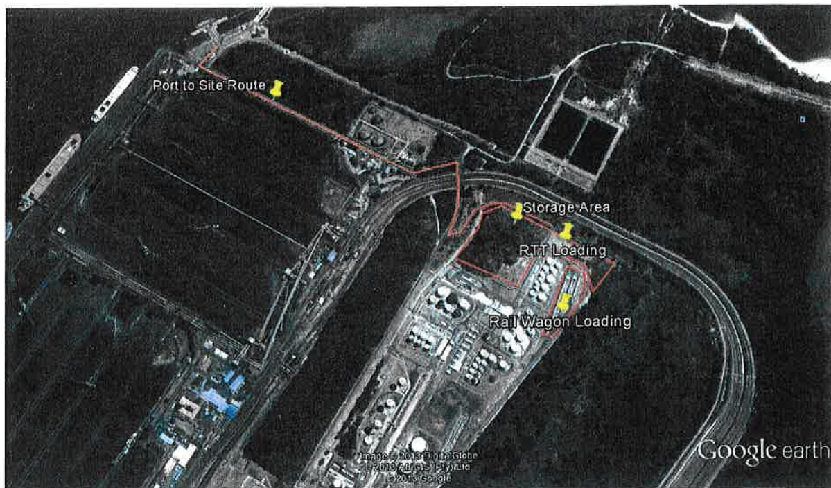
IVS Richards Bay aerial photo indicating new LPG area
